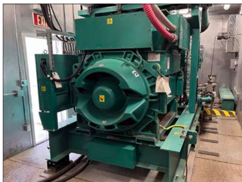
Cummins Natural Gas Generator Set QSK60 Series Engine Model C1400 N6C Mfr. 2018
